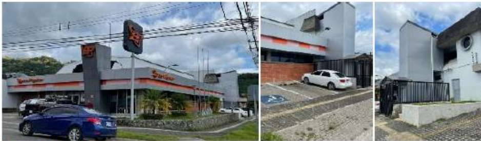
Fachada principal BPT Neilly
